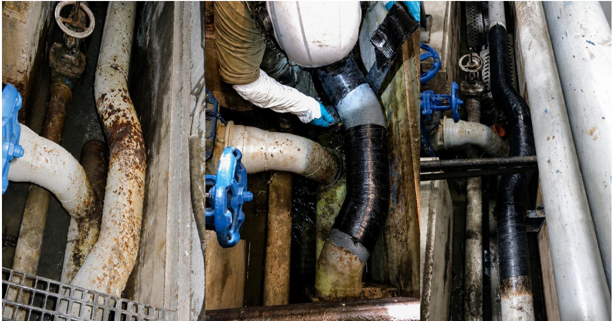
Composite wrap system applied to leaking pipeline. Image credit: Protecmo
